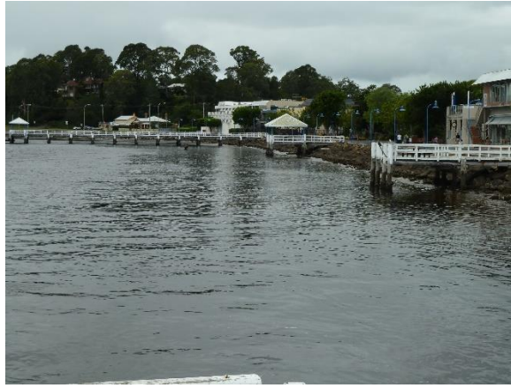
Multi-use Pontoon (A) Site. Wharf in foreground.
