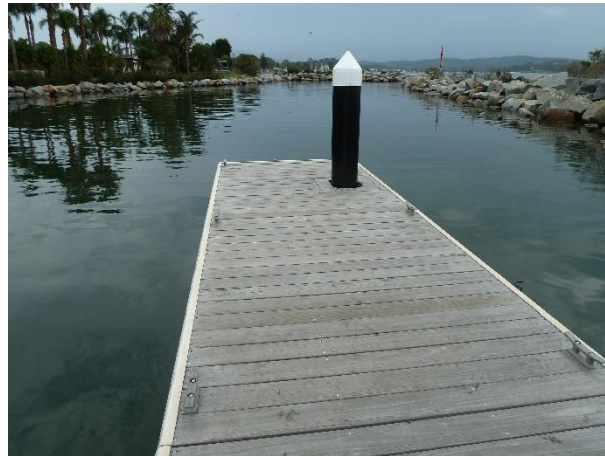
East side boat pontoon at Hanging Rock Boat Ramp
